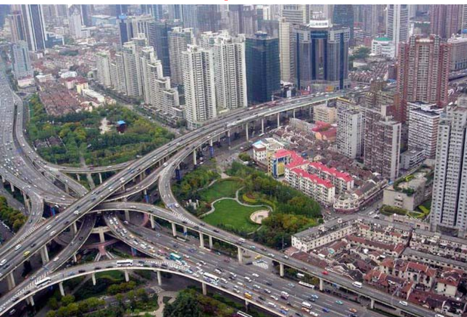
Puxi Viaduct, Šanghaj
