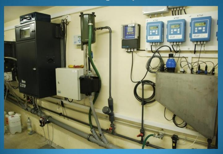
1st stage of chemical cleaning using aluminum sulphate.
